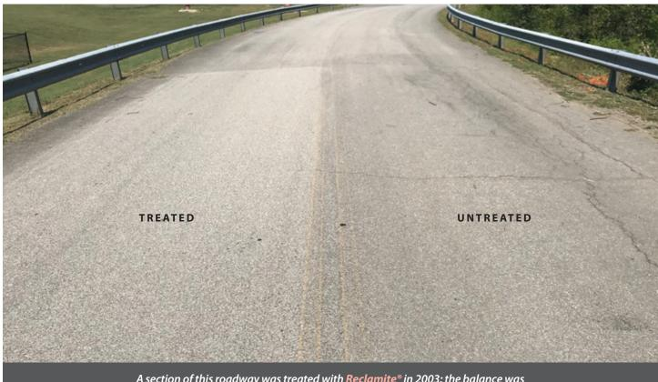
A section of this roadway was treated with **Reclamite**<sup>®</sup> in 2003; the balance was not. The photo was taken in September of 2019 — 16 years later!
