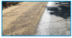
CRF® Restorative Seal is a cationic blend of asphalt and rejuvenator applied to pavements that exhibit more moderate deterioration including increased raveling, loss of aggregate and minor alligator cracking. Providing a "seal in depth," CRF® Restorative Seal is flexible and resilient, it does not harden or dry out.
