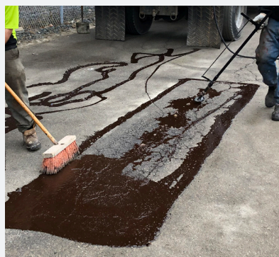
Cold Crack Filling & Paint Patching
