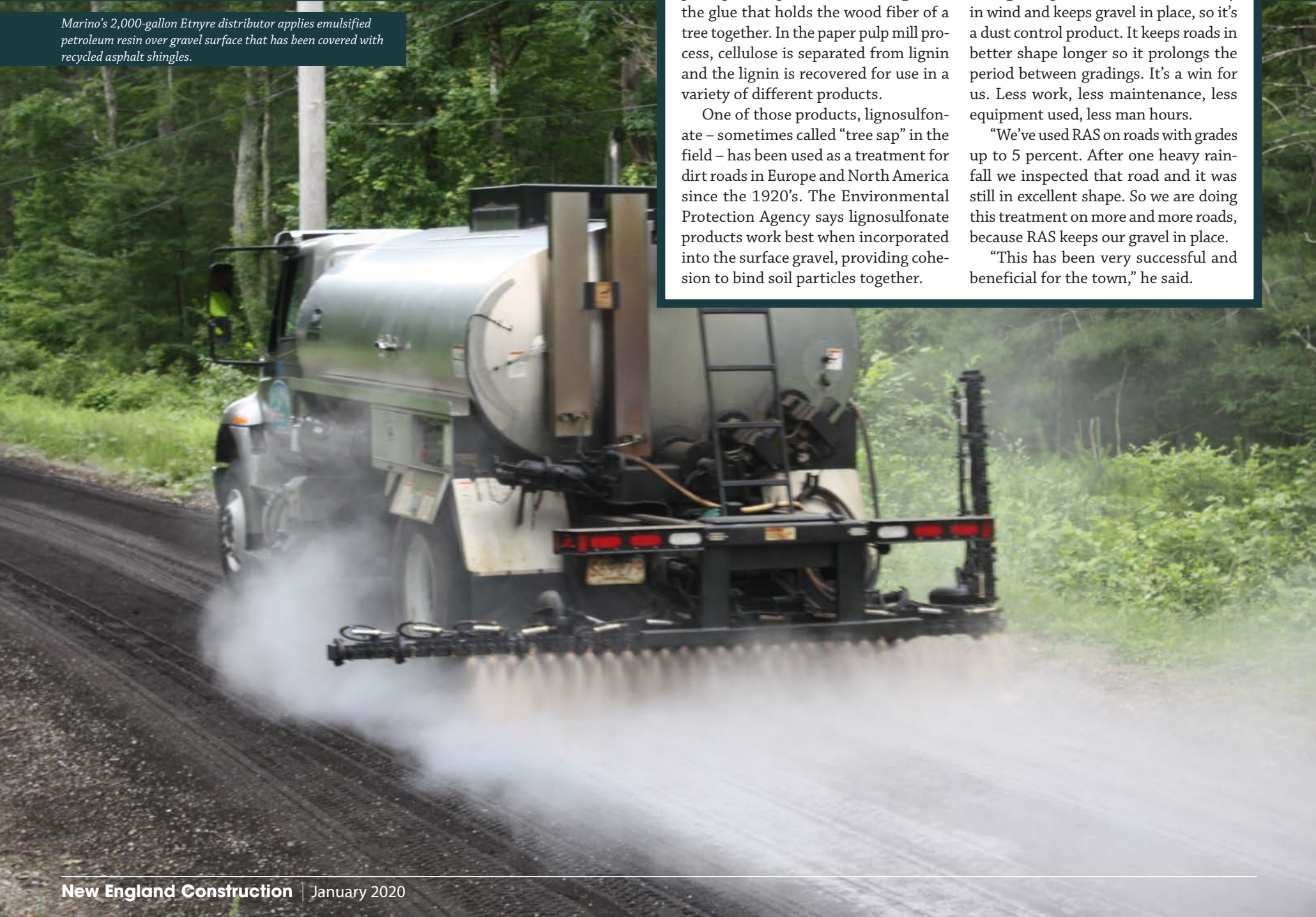
Felix A. Marino Co. Inc. International truck sprays emulsified petroleum resin to stabilize the road's gravel surface.
