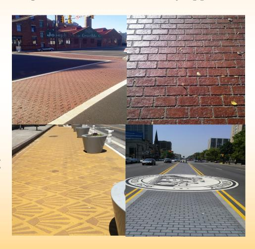
Can be applied to both asphalt and concrete pavement in a variety of colors, patterns and textures.
